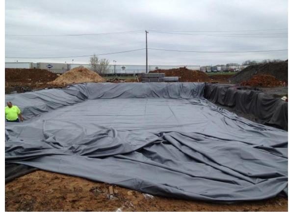
Image 2 – Impermeable liner installation
