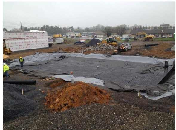
Image 3 – StormTank Module System installed
