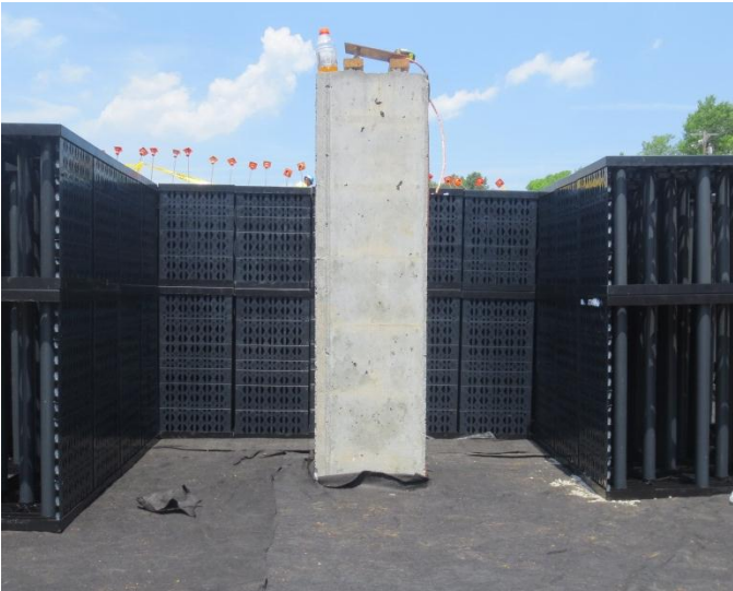
Image 3 – StormTank Modules Installed Around Foundation Column
