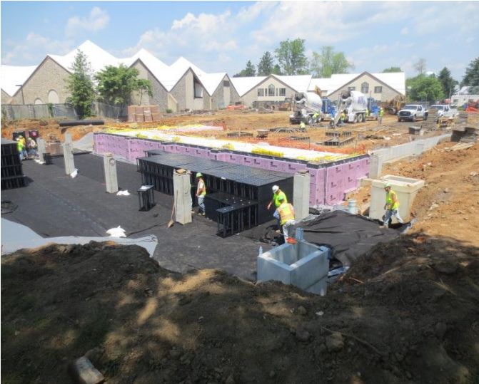
Image 2 – StormTank System Being Installed Along Building Foundation
